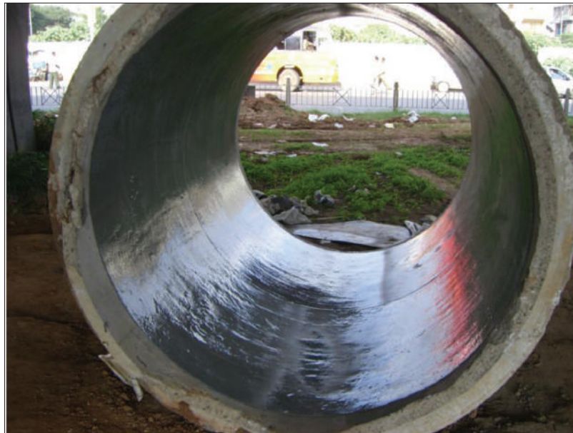
Figure 3.59 RCC Sewer pipe with protective coating
