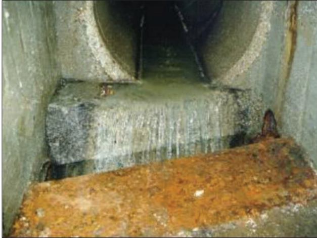
Figure 3.17 Typical floor level leaping weir
